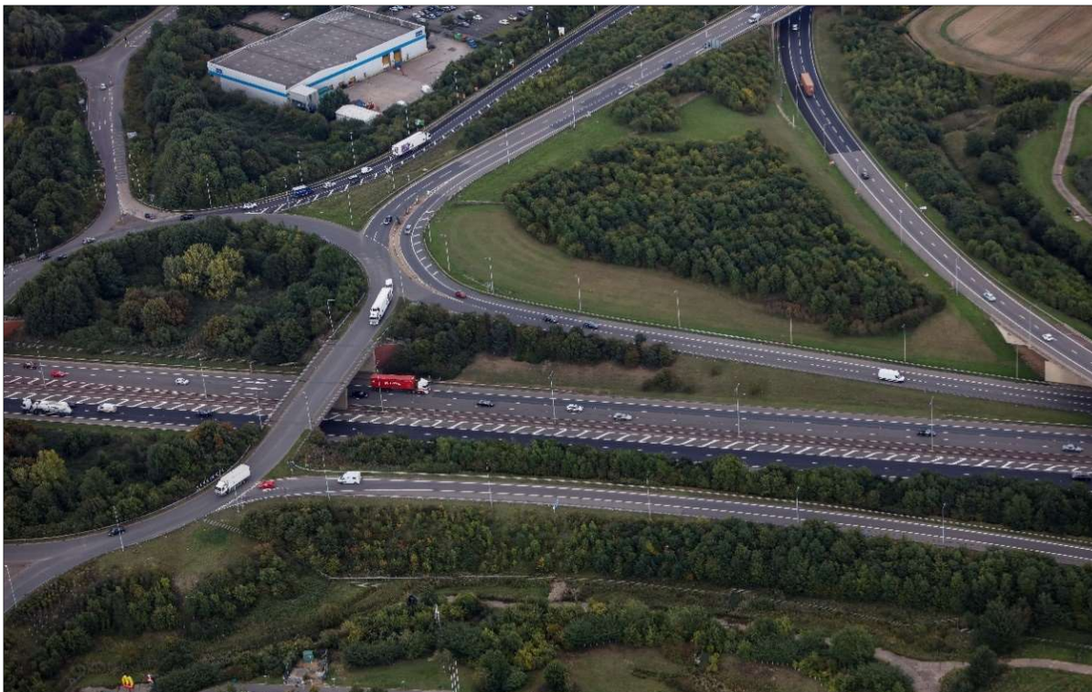
Figure 6.2: Junction 17 (A1M) Improvement (Post Scheme)
