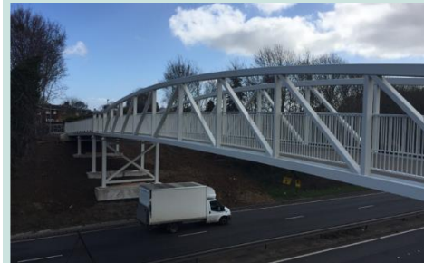
roundabout) of the Nene Parkway.
