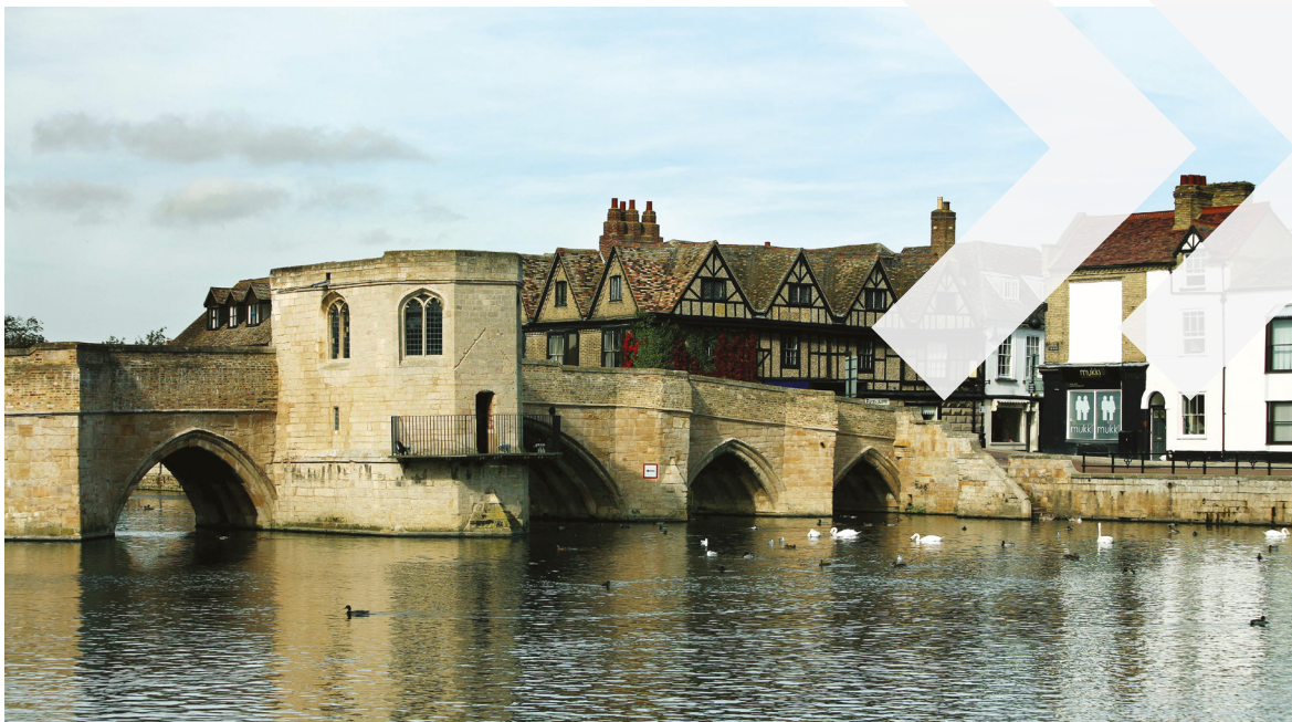
Bridge over the Great Ouse River in St Ives
