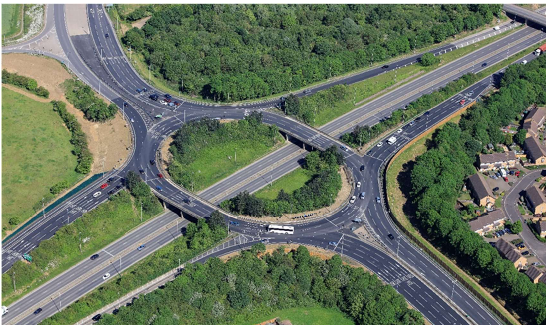
Junction 20 Improvement (post scheme)
